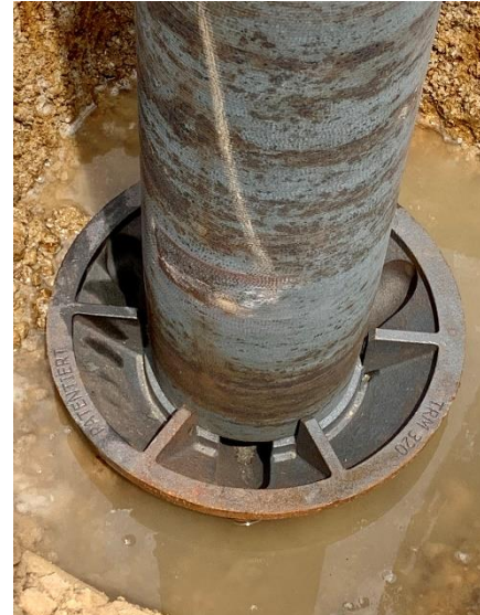
Figure 4. Conical shoe with grouting ports
