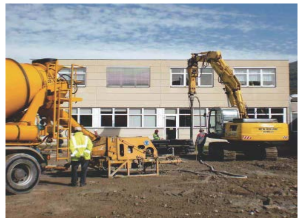
Photo 3 Driving Grouted Ductile Iron Piles
