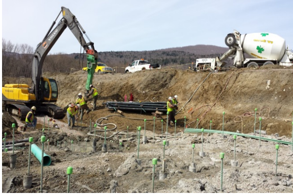
Photo 8 Driving Friction Piles in Waterbury Vermont. Note the variation in grades.
