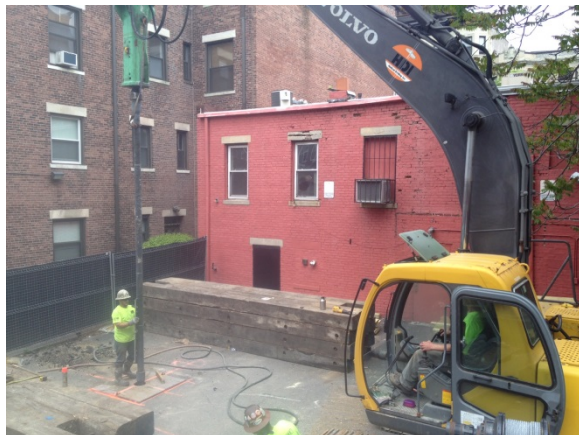
Photo 1 Driving a 170 foot long test pile in Boston
