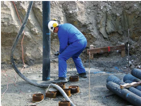
Photo 5 Cutting of a driven pile with a grinder
