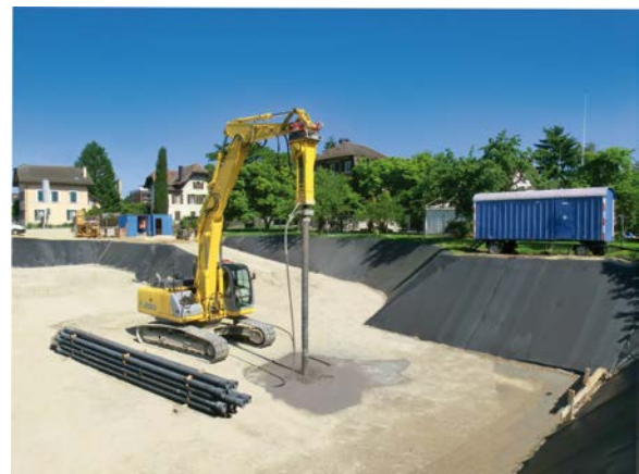
Photo 2 DIP driving operation on a flat site
