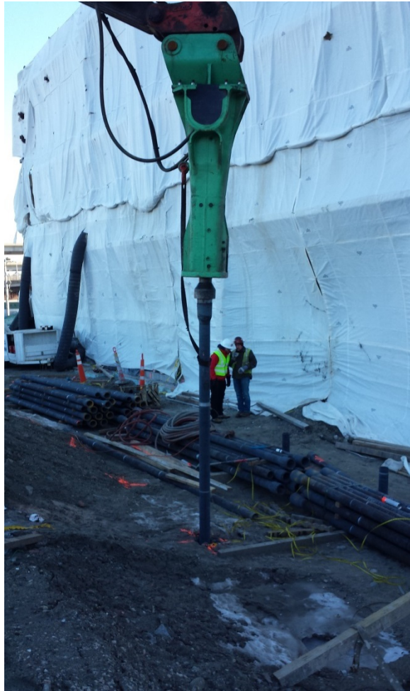
Photo 6 Driving End Bearing Piles at North Point
